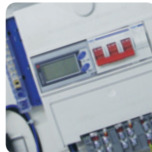
Metering fitted next to incomer within board
