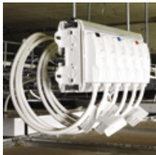
Figure 5 - Prefabricated wiring system using flexible cable
